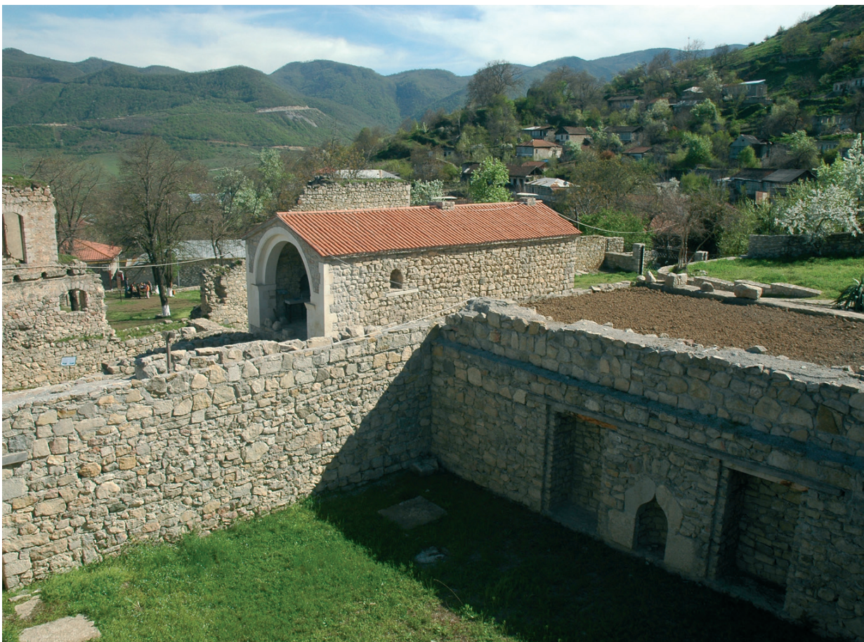
ill. 27 The general view of the melik mansion of Togh after the excavations and restoration.
